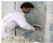
Step-2 Filling plaster material
