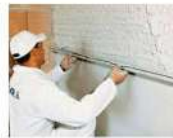
Step-3 Flatten the Plaster
