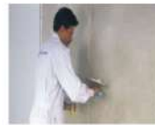
Step-4 Thin slurry coat for finishing
